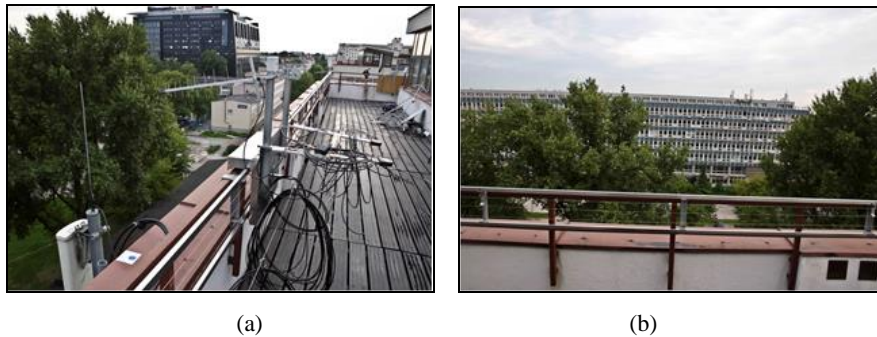
Fig. 1. The experiment description: The antenna on the trolley (a); the field of view (b)
